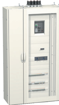
Power distribution switchboard.
